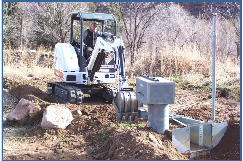
Alan Halley with Northern Water, works to install the Parshall Flume and uses an excavator to create a small trench behind the flume for controlled runoff and sample collection
